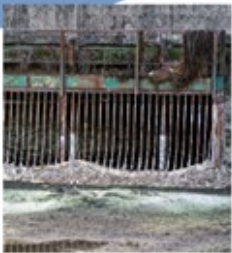
In-line Trash Nets or Screens Placing a trash net, screen, or other type of grate in the direction of flow captures trash that would otherwise flow past.
