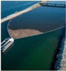
Floating Booms Floating booms installed on the water surface are typically anchored and collect trash while water flows past and underneath.
