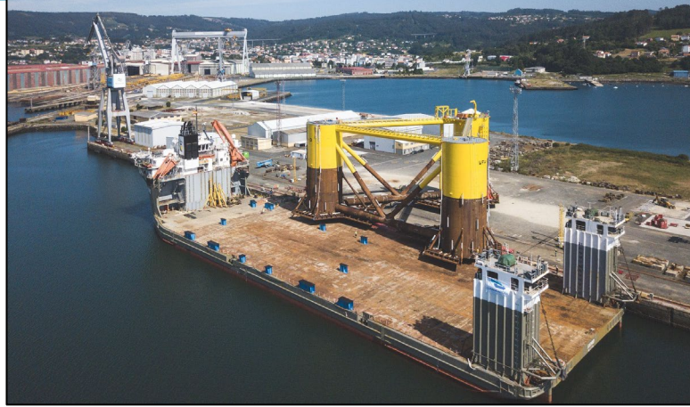
2) Loadout onto semi sub
