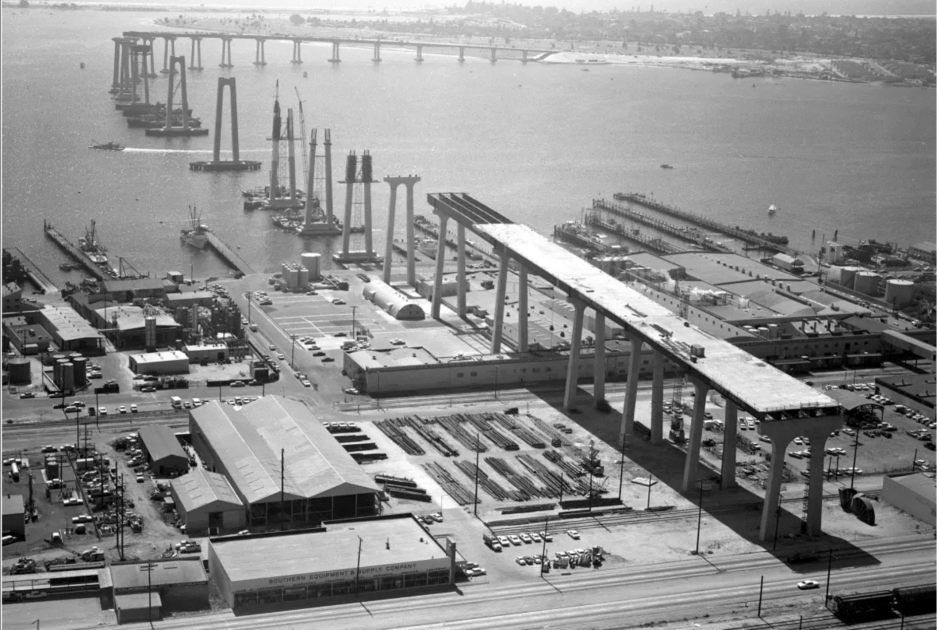
The Coronado bridge under construction in 1968
