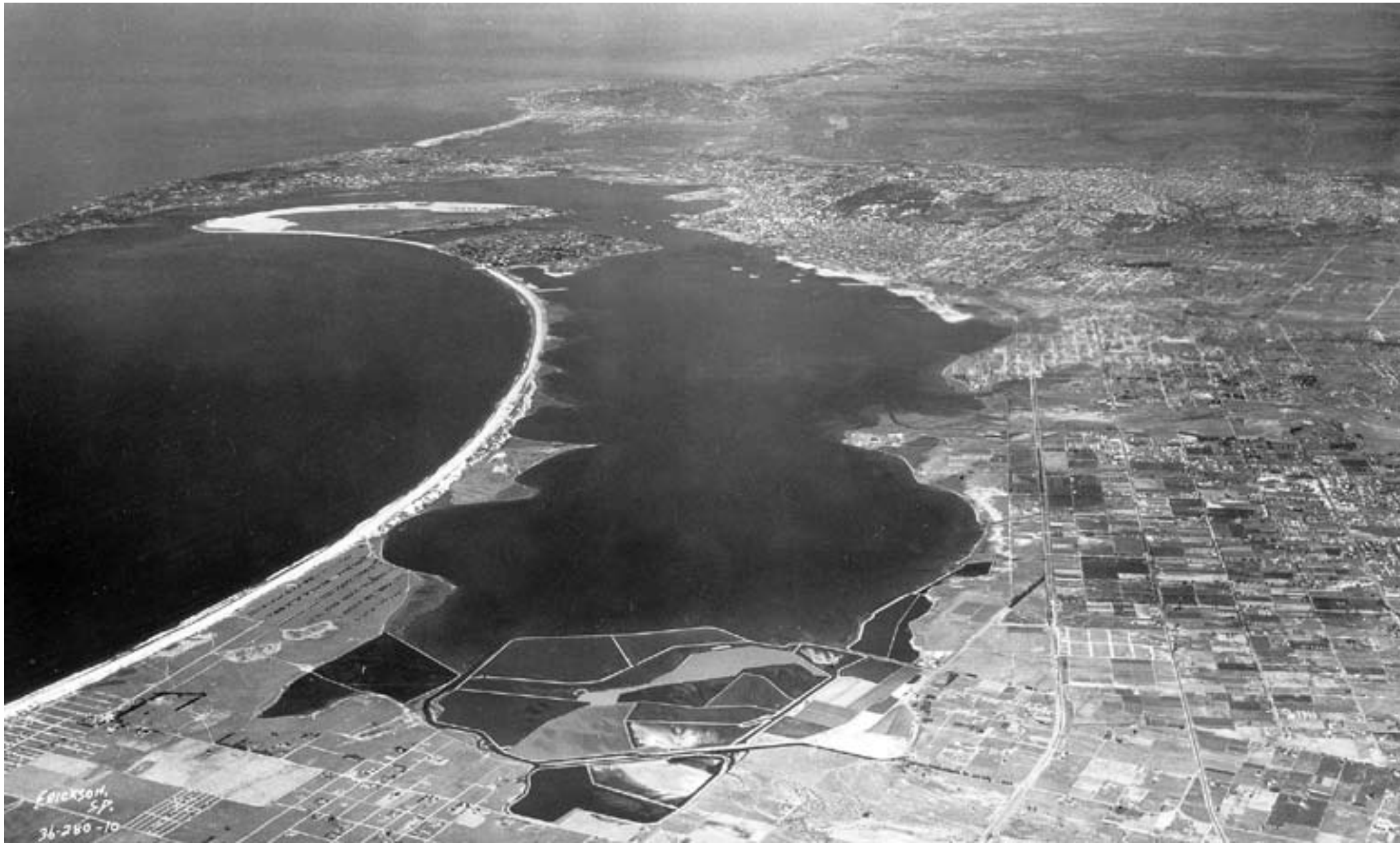
1936 San Diego Bay looking northwest
