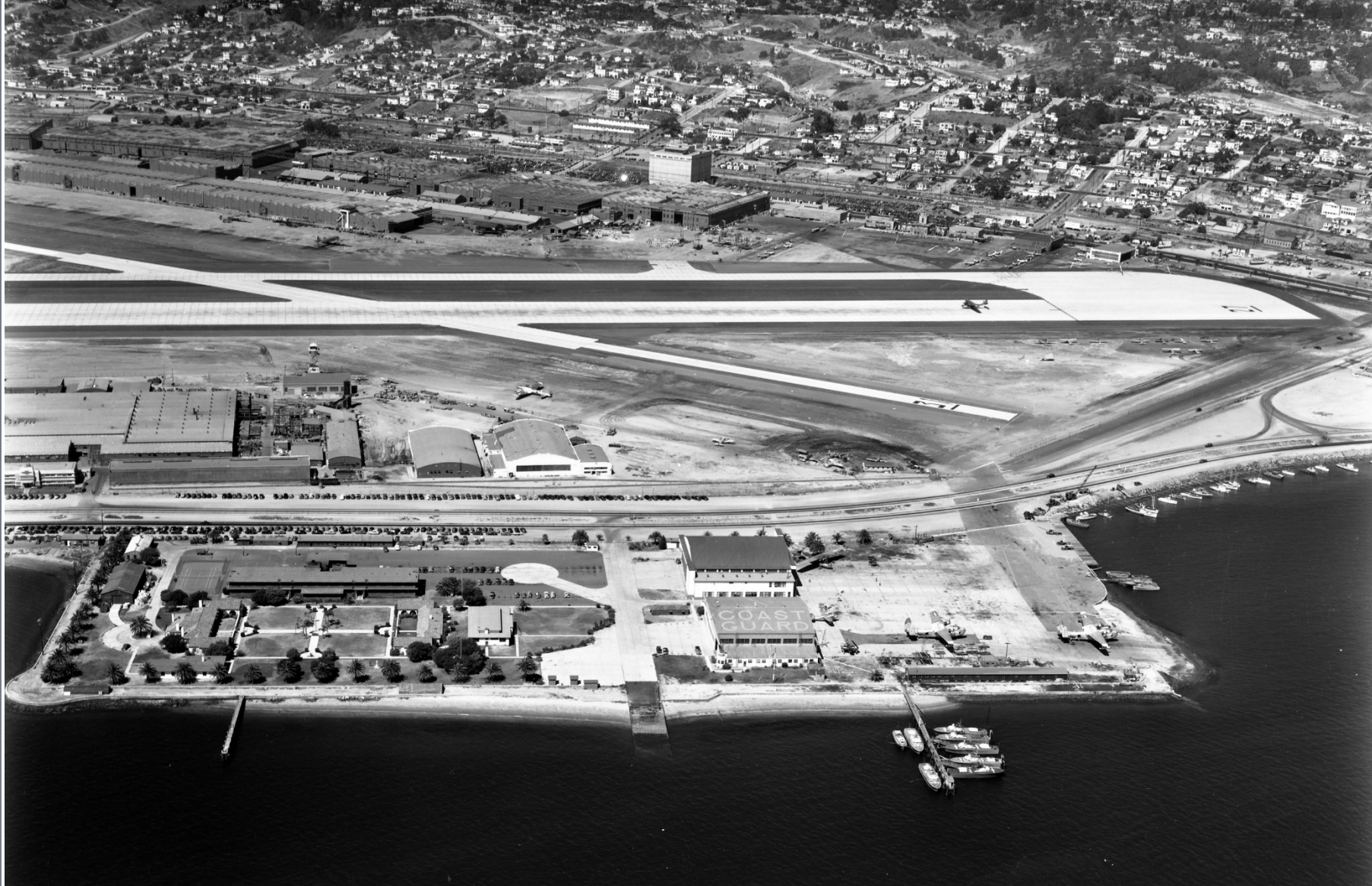
1946 Dredging San Diego Harbor around Lindbergh Field Airport
