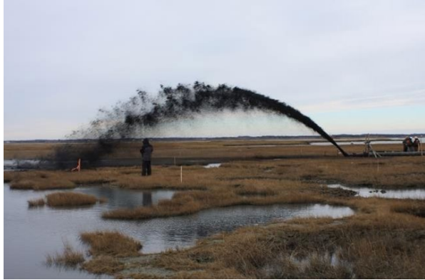
“Thin” Layer Placement (Sediment Enrichment) Avalon NJ (2014 and 2016)
